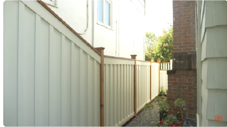
Hardie and wood frame (Fire Safe Marin)
