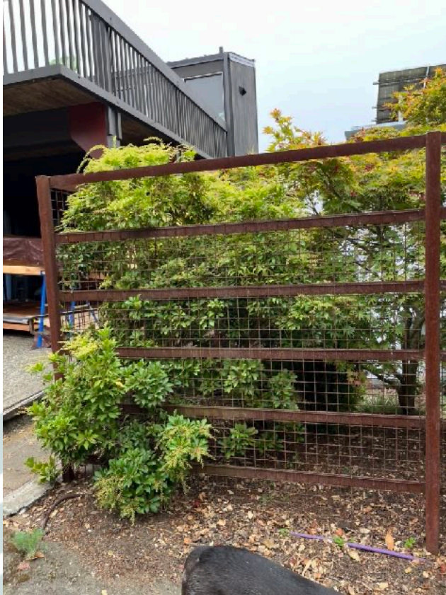
Steel frame and hog wire
