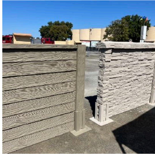
Pattern formed concrete
