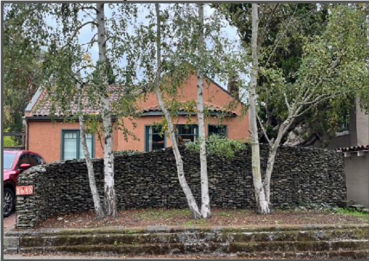
Gabion Wall in Kensington
