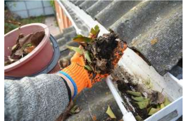
Regularly clean roofs and gutters!
